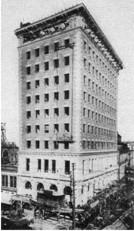
Union Bank, Winnipeg. Under construction, 1904
